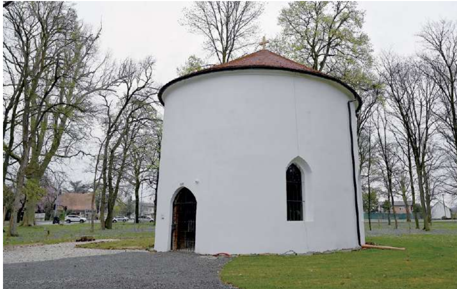
Fig. 2 The burial chapel has withstood despite poor maintenance over time and was restored in 2021 as part of the Living Heritage project (LAS programme) with the financial support of the Municipality of Murska Sobota (photography by Tajda Benko).
