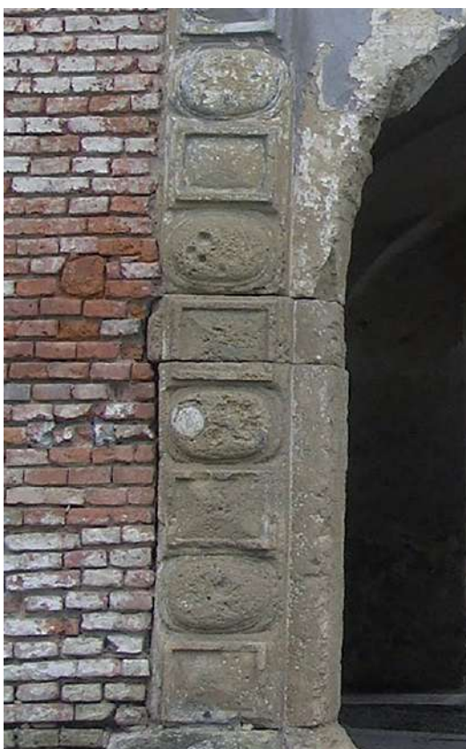
Fig. 6 Photograph of a single decorative field of the main portal of the Rakičan mansion prior to restoration, showing the stone structure and the base of the portal with an older grey coloured coating (photography by Tajda Benko).
