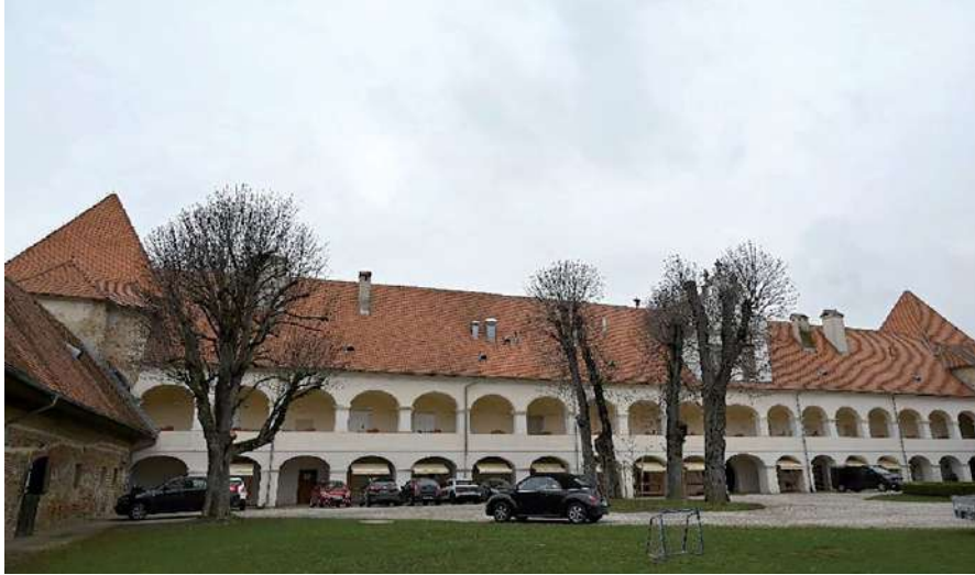
Fig. 9 The arcaded covered corridor with cross arches in the Rakičan manor, which provides access to various parts of the manor, including in bad weather (photography by Tajda Benko).
