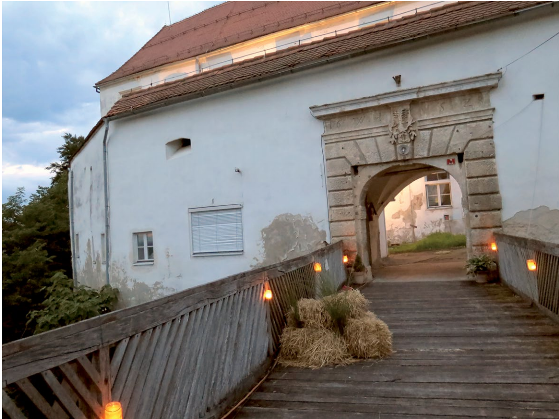
Fig. 7 A photograph of the entrance to Cmurek Castle in Trate (source: https://www.seviqc-brezice.si/trate-grad-cmurek.html ). Given the way the stone portal and the system of lifting doors are designed, a parallel can be drawn with the portal at Rakičan Manor, where a similar gateway marks the entrance to the manor. It can be affirmed that the knowledge was transmitted and that, in all probability, the builders of the portal were from the same school or workshop, in spite of the fact that Cmurek Castle belonged to the Austrian part of the monarchy and Rakičan Castle to the Hungarian part.
